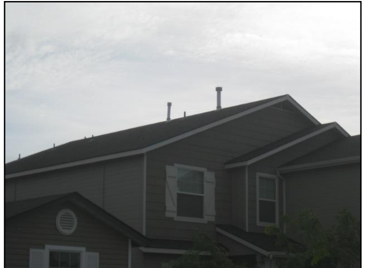
2. Asphalt shingles
