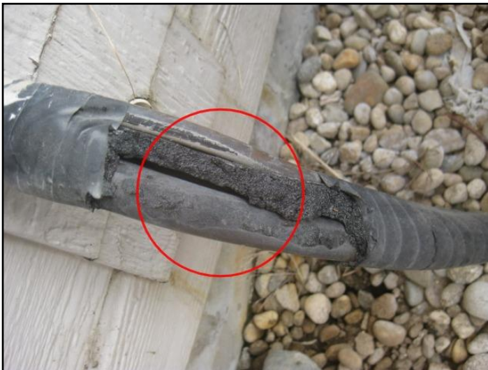
29. Missing insulation
