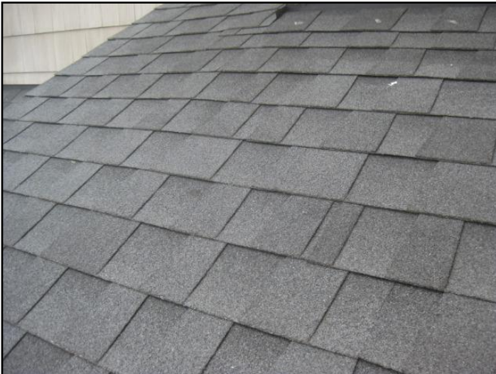
3. Asphalt shingles
