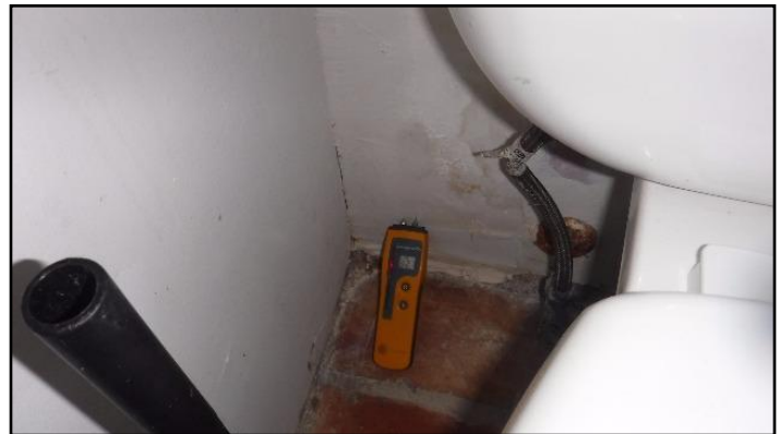
10. Water damage
