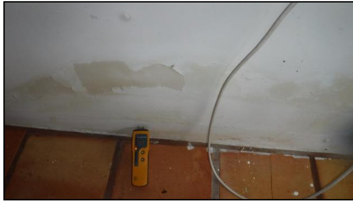
8. High moisture reading
