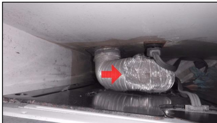
15. Dryer vent obstructed
