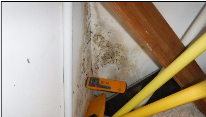
9. Water damage
