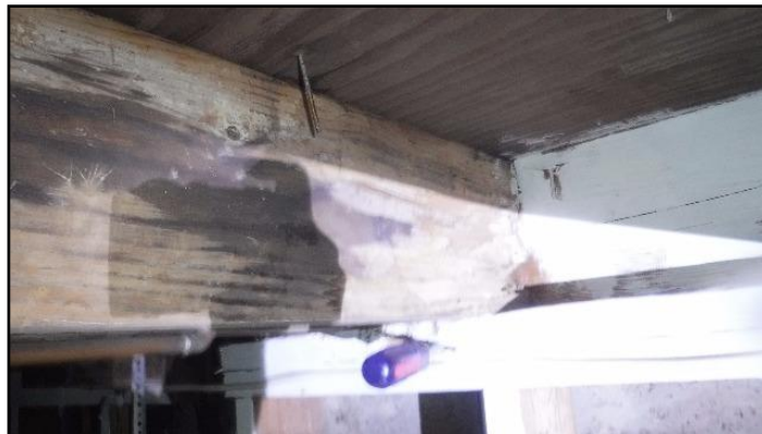
2. Rot or insect damage
