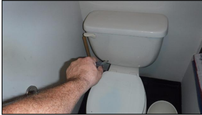
6. Flush mechanism inoperative
